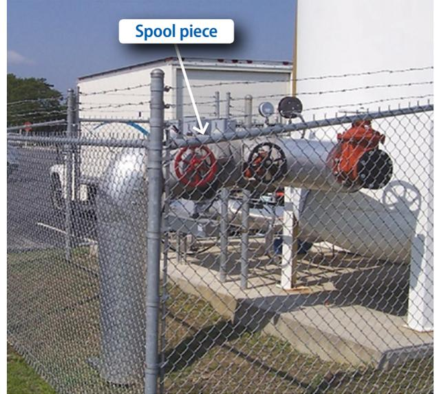
For accessible explanation of these two images about spool piece to be removed when not in use, and location of spool piece see [Appendix G](#).
