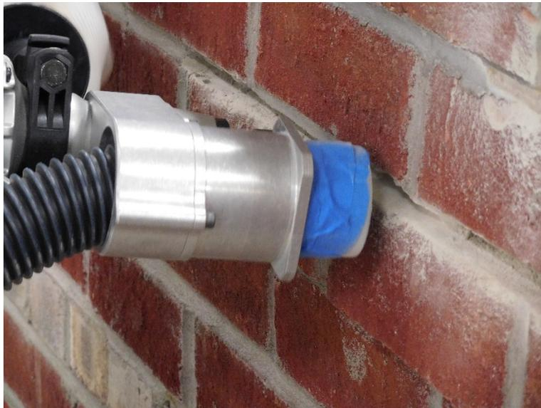
**Figure 5 – Hood close to work surface**
