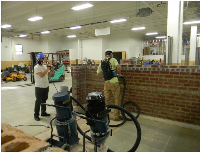
Figure 4 - Pre-separator (left) and vacuum cleaner (right) (NIOSH photo)
