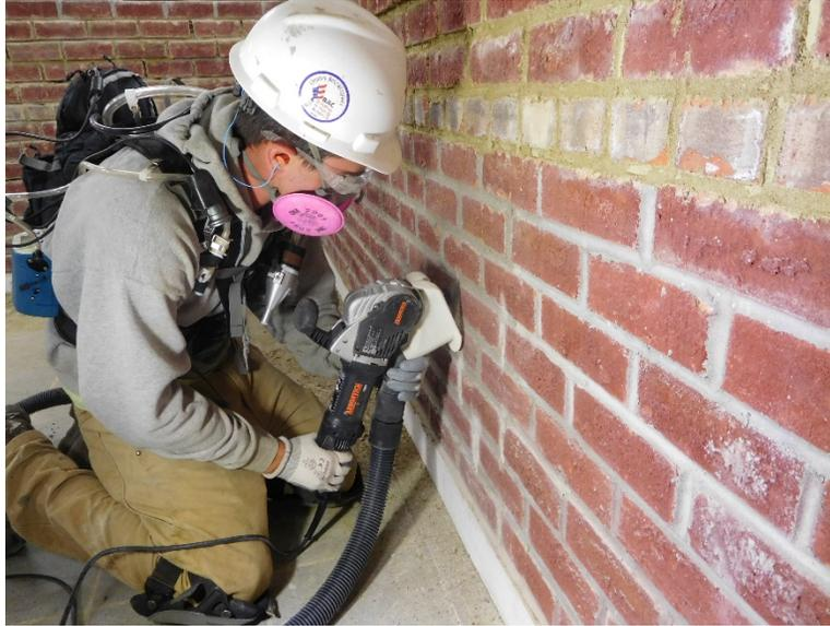
**Figure 2 - Saw with modified hood (NIOSH photo)**
