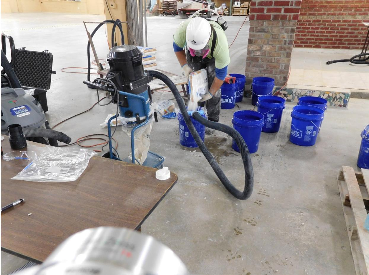
Figure 2 – Adding thinset mortar to bucket (NIOSH photo)
