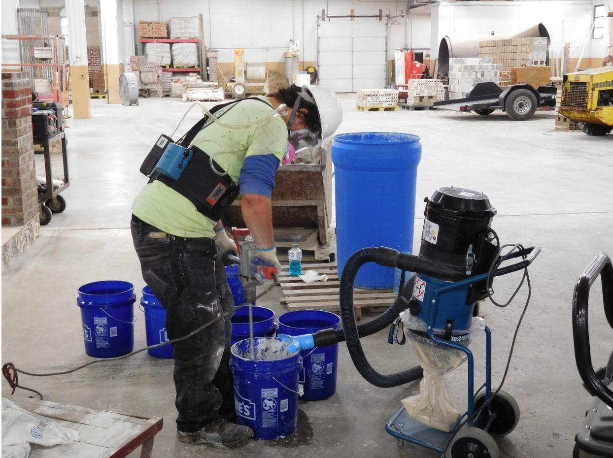
**Figure 3 - Mixing thinset mortar and water with drill (NIOSH photo)**
