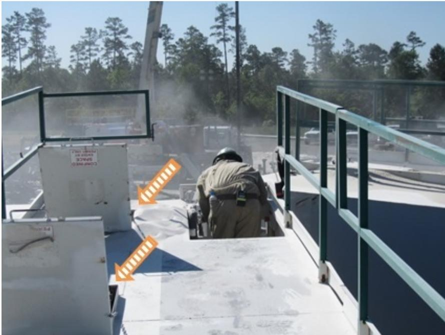
Figure 2. Sand Mover Operator at his work station on top of a sand mover, with arrows pointing to the open thief hatches. Photo courtesy of Eric Esswein, NIOSH.
