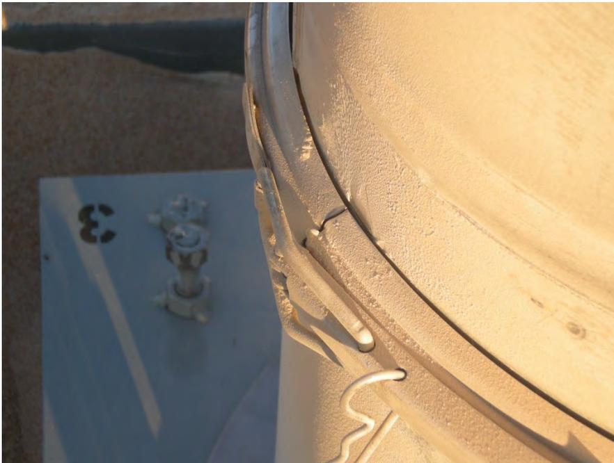
**Figure 20. Dust leakage visible at the band clamp connecting two sections of ductwork on the mini-baghouse. Photo courtesy of Mike Gressel and Jerry Kratzer, NIOSH.**
