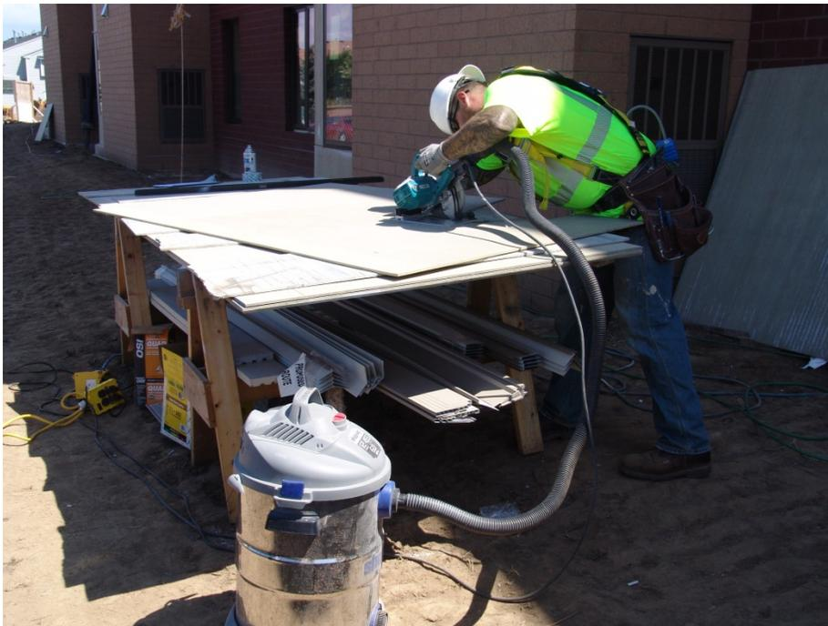
**Figure 2 – A worker (cutter) cutting fiber-cement siding using a dust-collecting circular saw that was connected to a shop vacuum. Photo courtesy of NIOSH.**
