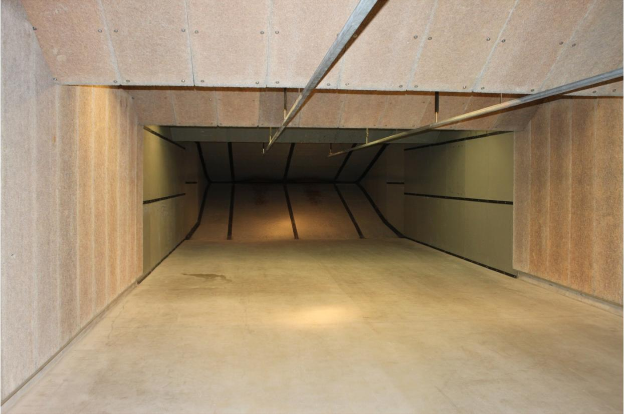
**Figure 13. Acoustical treatments to walls and overhead panels at the WPAFB indoor firing range**
