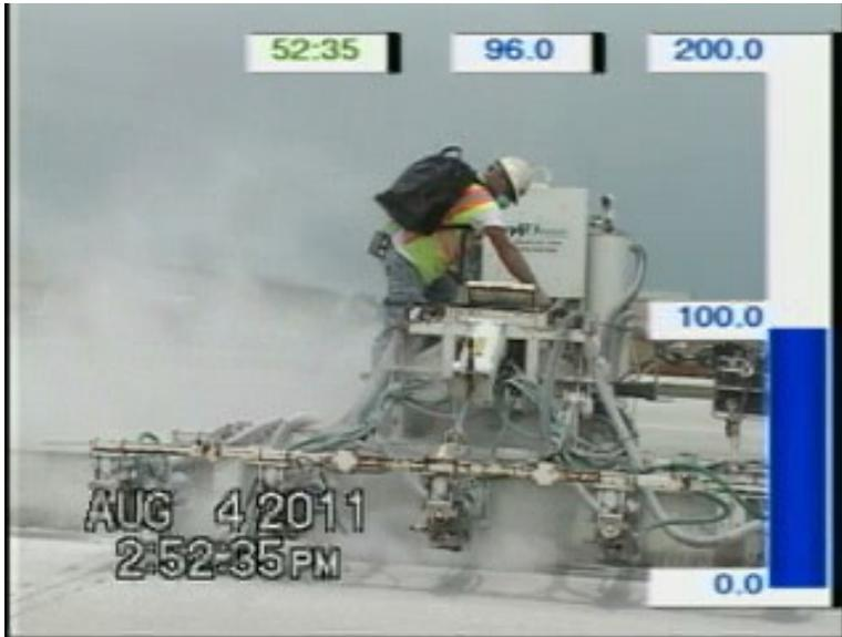
Figure 11 - Purging the Dust Collection System Produced a Spike in Respirable Dust Exposure
