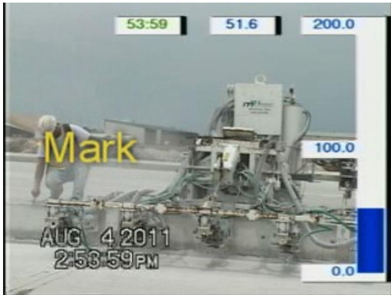
**Figure 10 - Marking the Concrete During Drilling Produced a Spike in Respirable Dust Exposure**
