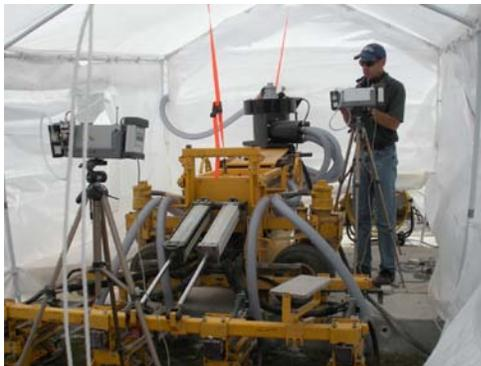
Figure 2 - The dowel-pin drill inside the tent
