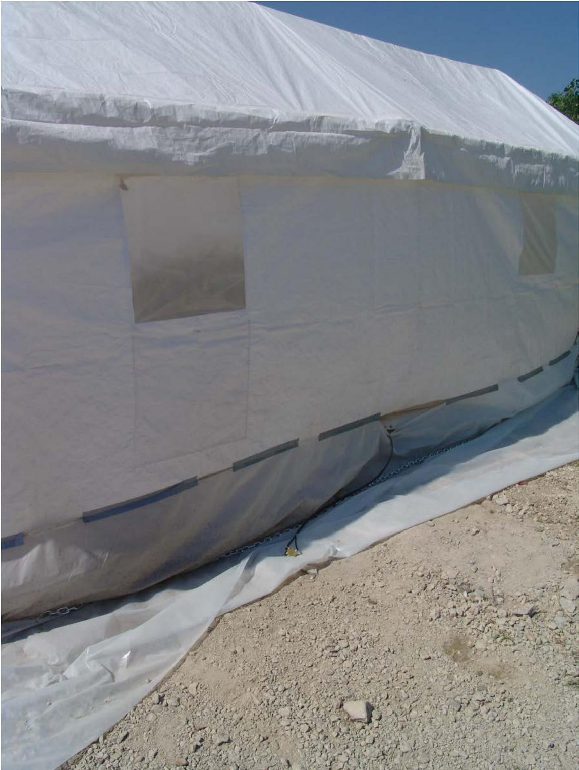
Figure 3: Chain and Sheeting Hold Tent to Ground. Note the Remote Starter Switch.
