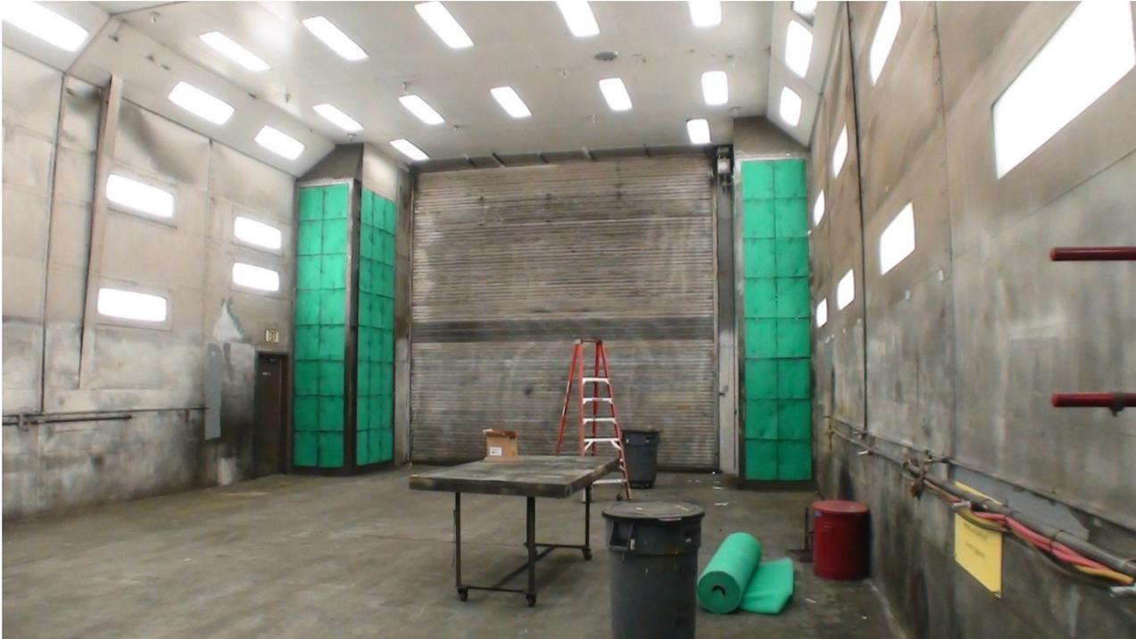
Figure 5. The Fort Lewis helicopter painting hangar. The exhaust filter columns can be seen on either side of the hangar door.
