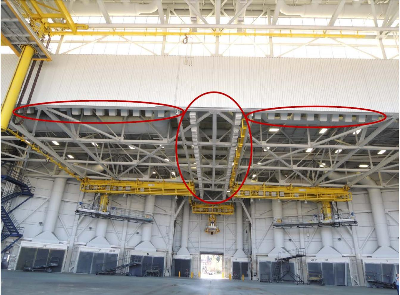
Figure 4. Photo of the JBLM corrosion control hangar. The eight large exhaust hoods are visible along the back wall, and the small square supply inlets can be seen on the ceiling (circled in red).
