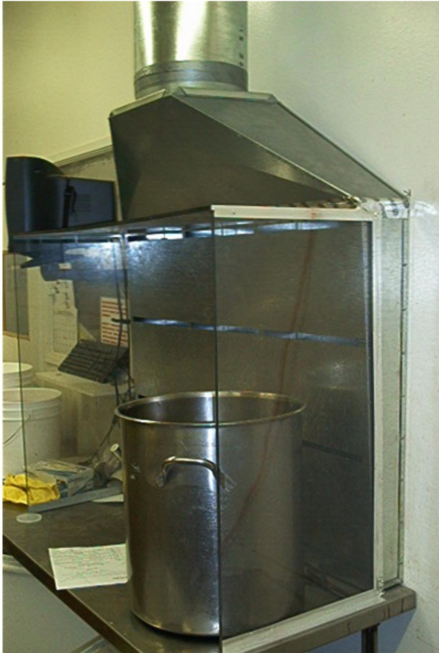
**Figure 3. Ventilated booth-type exhaust hood.**
