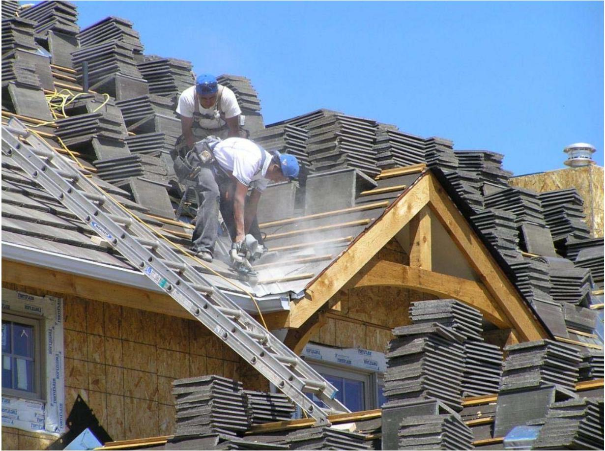
Figure 3. Roof arrangement while installing tiles.
