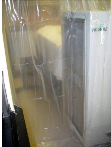
Figure 16. Photograph showing the freestanding HEPA filtration unit positioned between the two inner isolation zones. The edge of the curtain was sealed to the HEPA unit, and a vertical partition equally divided the inlet to prevent migration between the two inner isolation zones.
