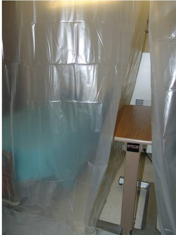
Figure 28. Photograph showing HEPA exhaust corridor, with tray table in place to resist curtain pull into the corridor.
