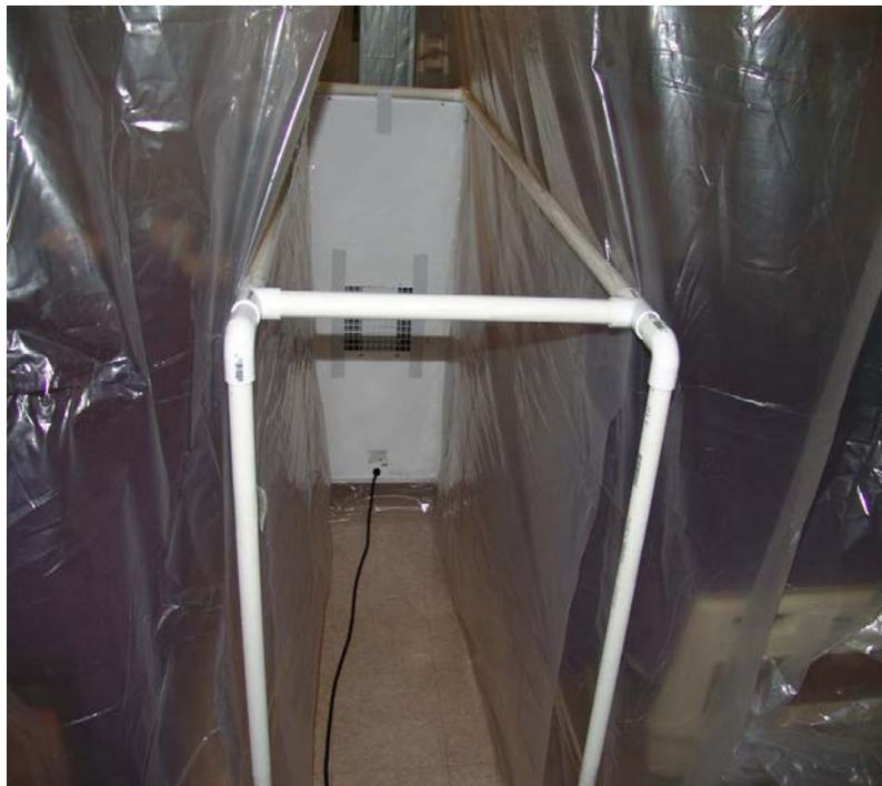
Figure 34. HEPA exhaust corridor with exhaust tunnel in place, relieving the isolation curtain from the inward pull created by frictional drag and induced air movement.
