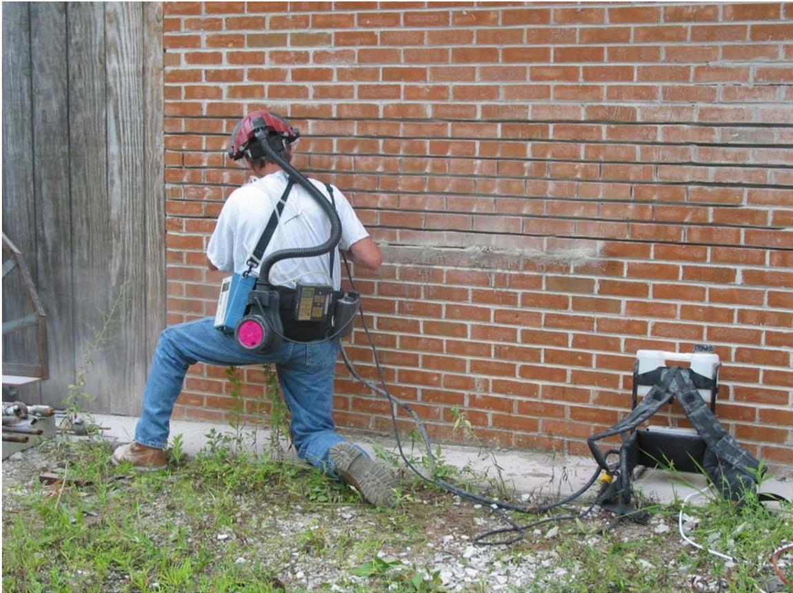
Figure 8: Mixture of mortar, water and brick dust on wall following use of Bronco control
