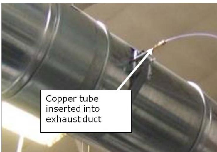
**Figure 13: Copper tube to sample tracer gas from exhaust duct**
