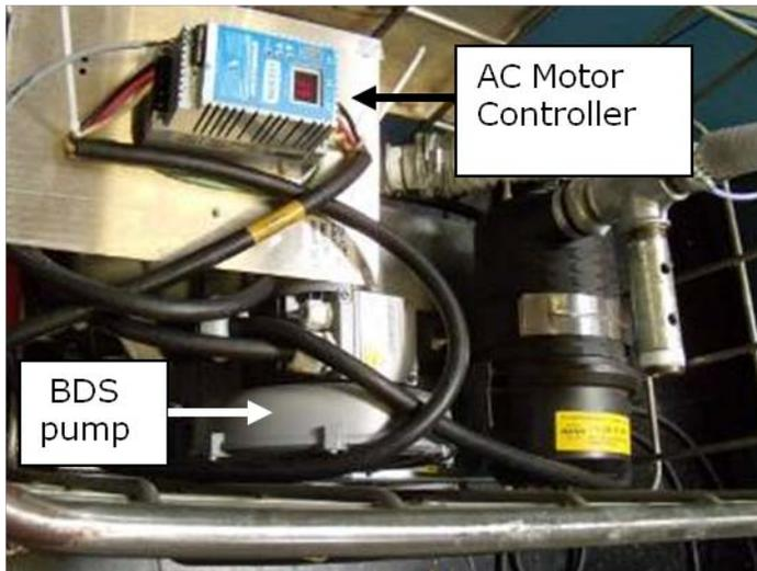
**Figure 11: BDS simulation pump**
