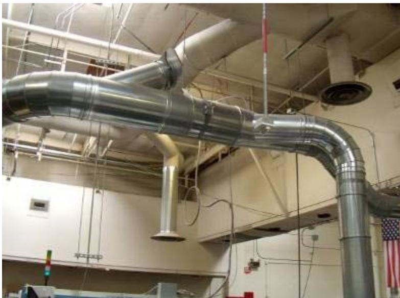
**Figure 9: General building ventilation supply diffuser locations**
