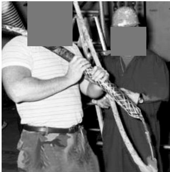
Figure 15. Cable Being Attached to Pull Rope
