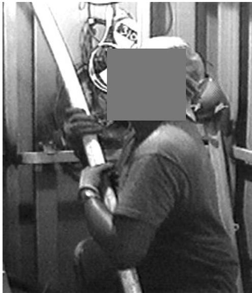
Figure 5. Cable Puller Crouching, Beginning to Push-Up 2-3" Diameter Cable
