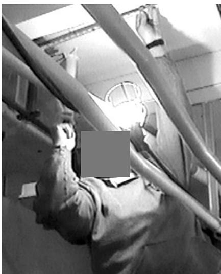
Figure 12 .Insulation Installer Measuring Insulation
