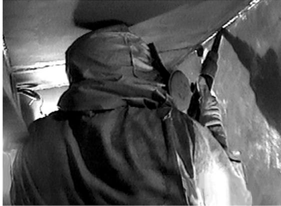
Figure 17. Tank Grinder Using Needle Gun Overhead
