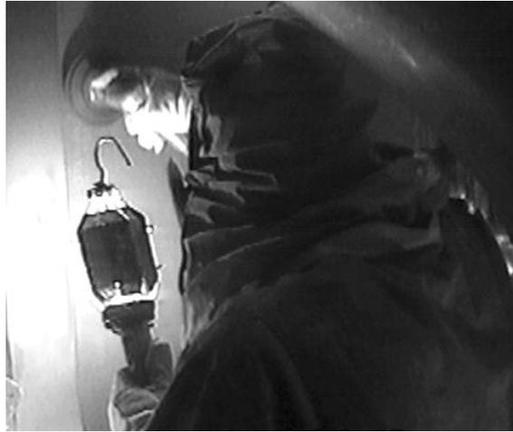
Figure 15. Tank Grinder Using 5-Inch Offset Grinder
