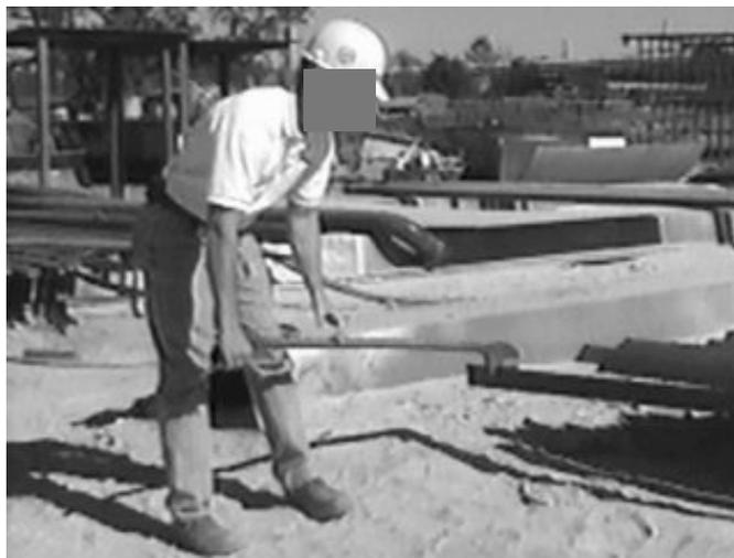
Figure 3. Gator Bar Worker Flipping Angle Iron from Side with Gator Bar
