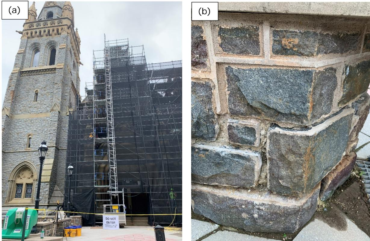
**Figure 1 – (a) the stone wall building under renovation; (b) a closeup view of the wall where tuckpointing was to be conducted for the building renovation. Photos by NIOSH.**
