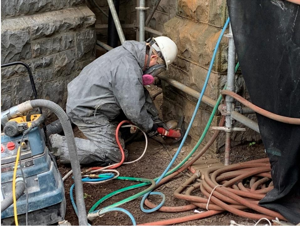
**Figure 2 – A bricklayer using a handheld pneumatic wet grinder with a diamond blade to cut a line in the middle of the mortar. Photos by NIOSH.**
