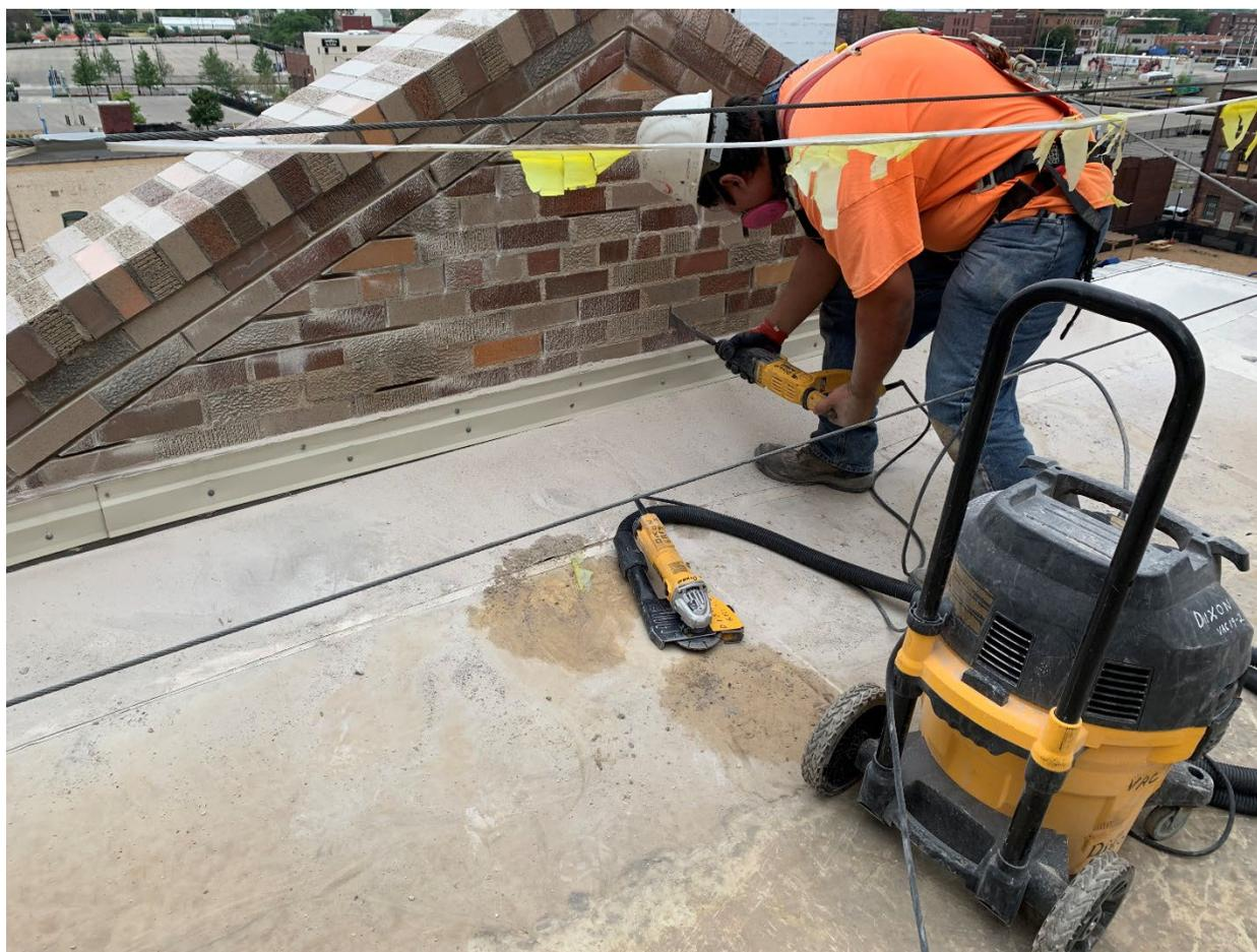
**Figure 3 – A power chisel without LEV and a dry grinder with a 10-gallon wet/dry vacuum cleaner providing LEV used for tuckpointing. Photo by NIOSH.**
