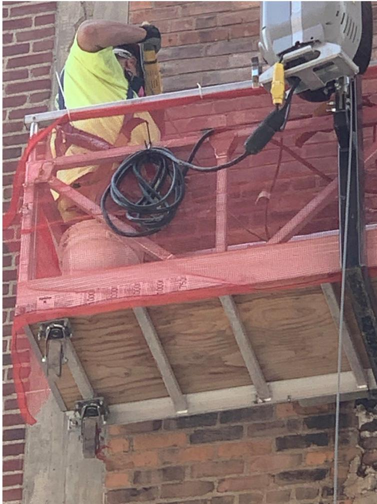
**Figure 2 – A bricklayer using a power chisel without LEV for tuckpointing. Photo by NIOSH.**
