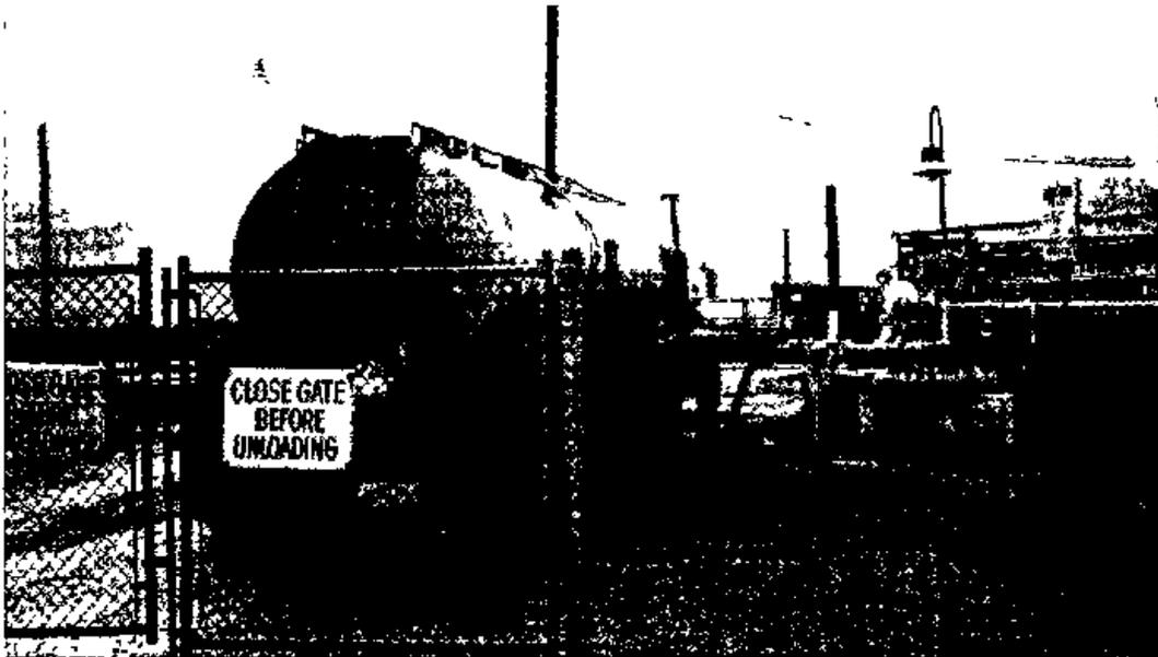
Figure 8. Methanol unloading area. Note gate and warning signs. Truck is in unloading process.
