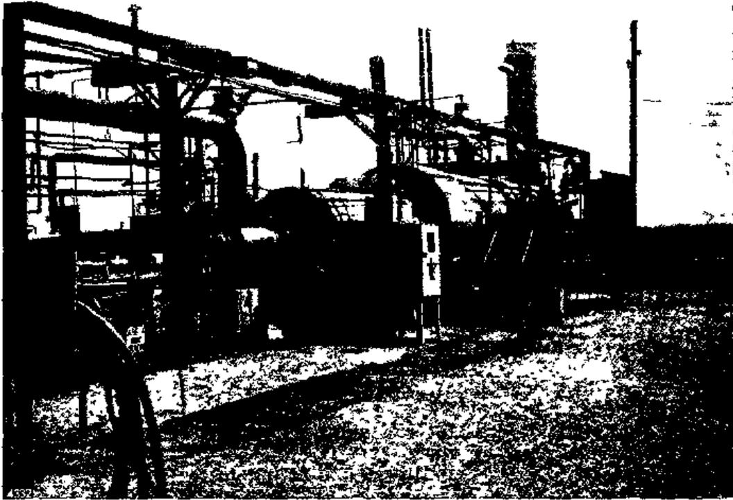
Figure 16. Waste heat recovery boiler.
