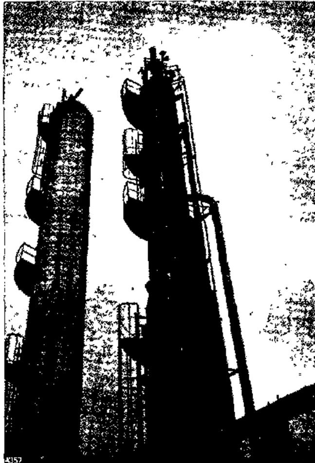
Figure 17. Absorber (right) and distillation column. Note exhaust line downstream of absorber.
