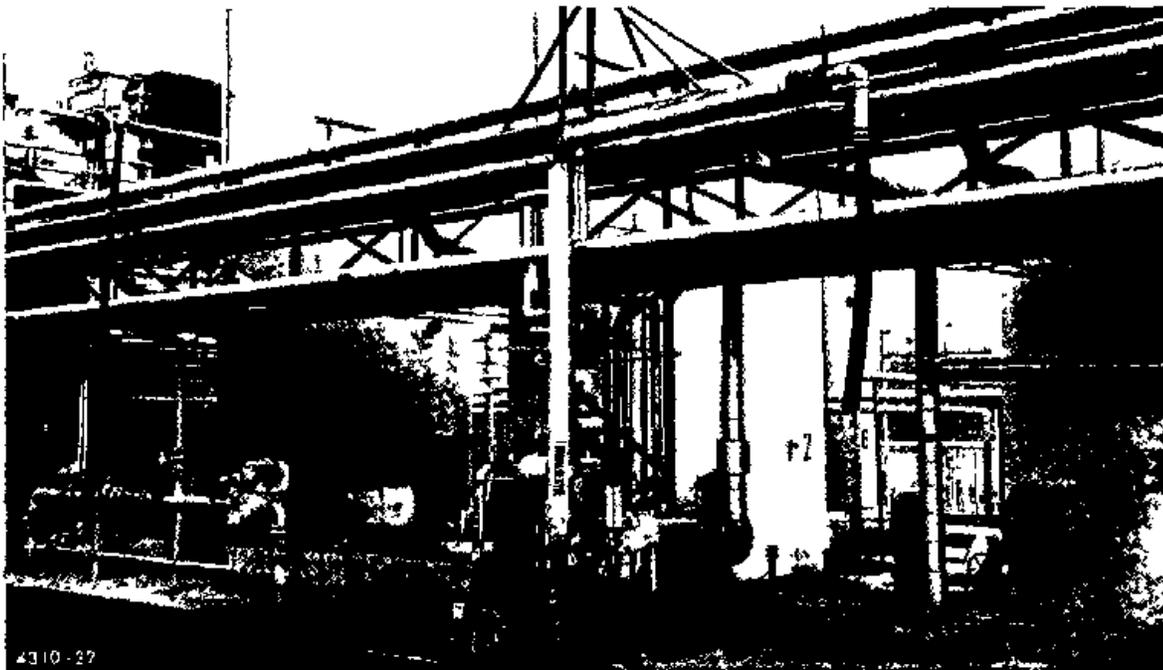
Figure 31 Formaldehyde tank truck loading area with swivel boom and flex-line loading spout and safety shower/eyewash station in background.
