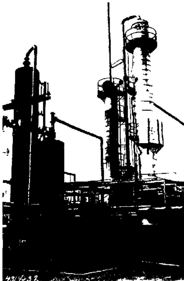
Figure 17. Production area, left to right - tall spray tower and short spray tower, packed tower with stack, distillation (stripper) column, air cooler and makeup water. Sample discard on right corner of cooler. Note diking.
