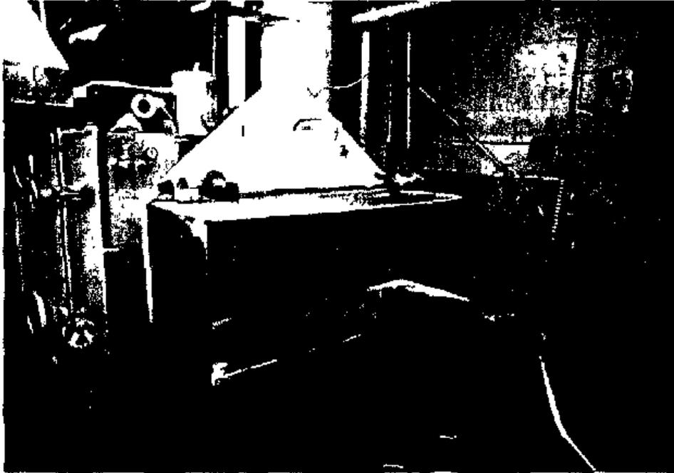
Figure 10 Three Sided Back Draft Slot Hood Over Loading Tray Station
