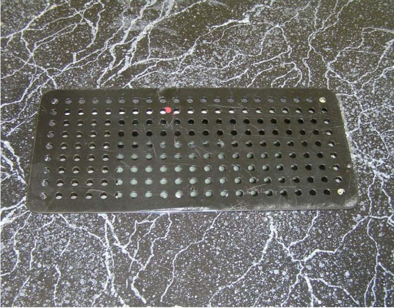
Figure 7: Downdraft exhaust hood built into the table
