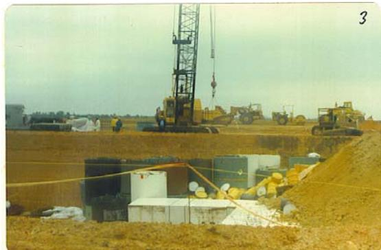
foam-uranium drums to Barnwell, SC, or Hanford, Washington disposal sites. The site photo shows NMI drums being dropped into a disposal pit. They had a long way to drop. When one of the drums was dropped a spark was generated which caused the drum to explode. I assumed this explosion was caused by accumulated hydrogen that pressurized the drum as hydrogen was released by the dissociation of water by the uranium.
