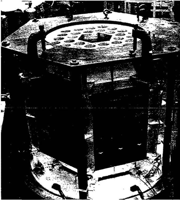
Figure 3-8. Parent core during construction (Thornton and Rothstein 1962).
