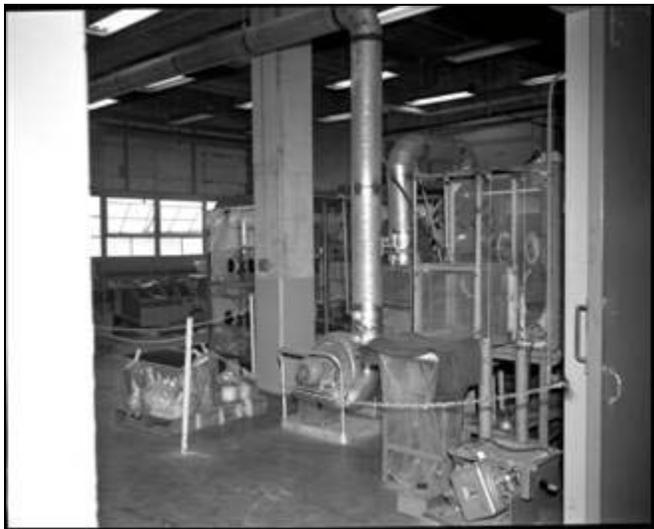
Figure 8. Containment ventilation equipment with HEPA filtration. Source: Coughenour (2009). The photograph is unclassified and does not contain UCNI.
