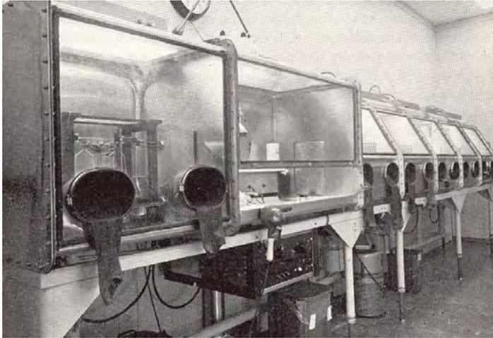
Figure 4 Plutonium gloveboxes at LANL's CMR facility<sup>(1)</sup>
