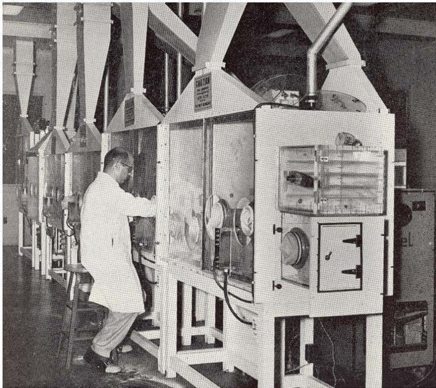
Figure 2 Plutonium gloveboxes at Chalk River<sup>(1)</sup>
