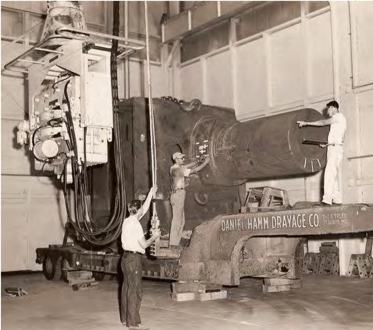
Figure 19. Betatron Radiography of the Axle of a Power Shovel Cast at GSI
