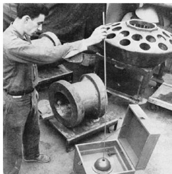
Figure 2. Source Being Removed from its Shield ("pig") (ORAU 1999)
