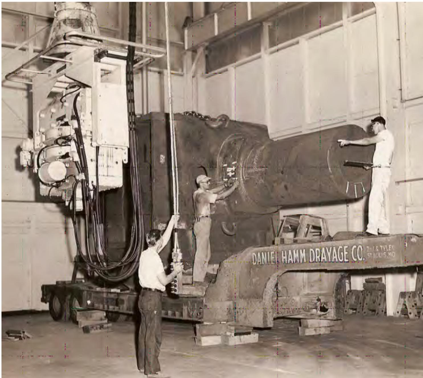
Betatron Radiography of the Axle of a Power Shovel Cast at GSI
