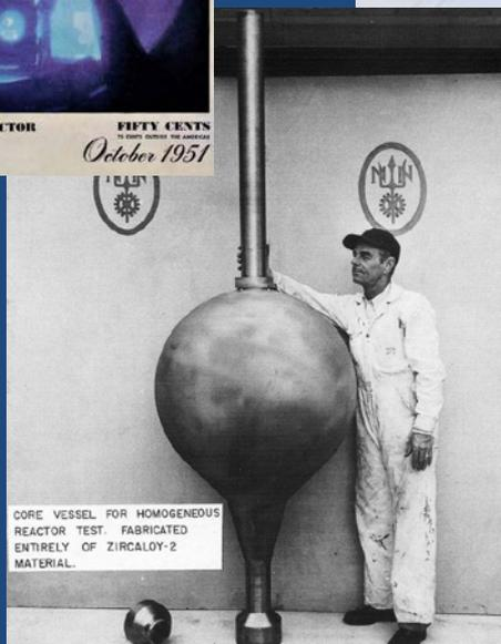
Homogeneous Reactor Vessel
