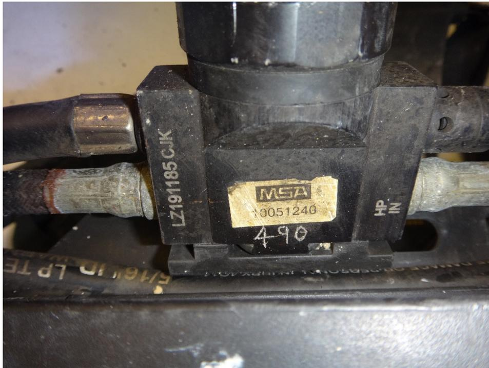
Figure 786: Side view of pressure reducer with labels
