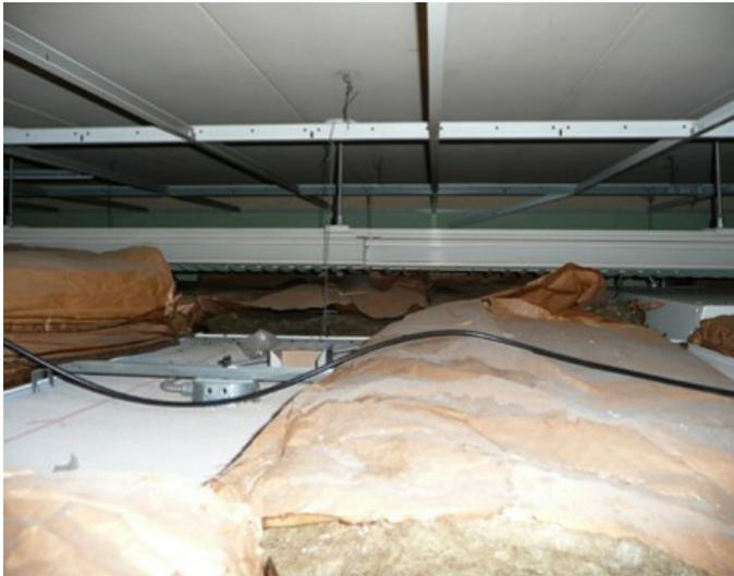
Figure A4. Dusty roll-faced insulation in plenum above classroom. Photo by NIOSH.
