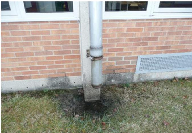
Figure A6. Broken and disconnected exterior roof drain outside classroom. Photo by NIOSH.
