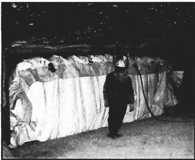
Figure 16.—Construction of seal in crosscut 2 showing vinyl bladder in place, but not yet filled.
