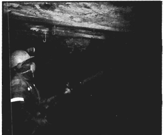
Figure 13.—Shotcreting of the spreader bar and hook assembly.
