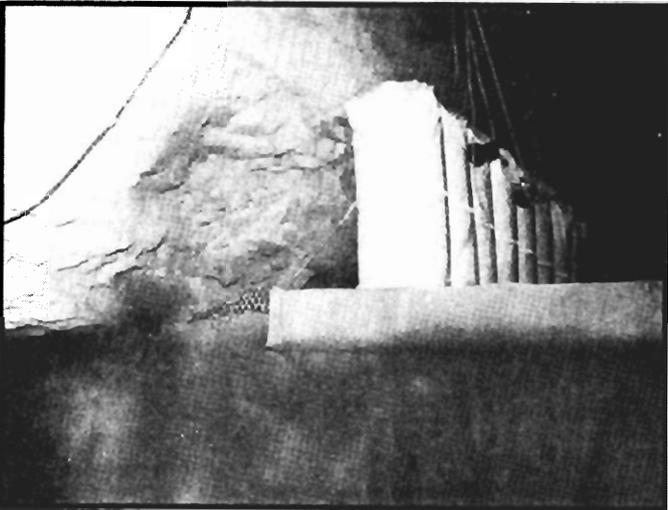
Figure 32.—Construction of wing wall along edge of overcast deck: end view of wing wall above deck.
