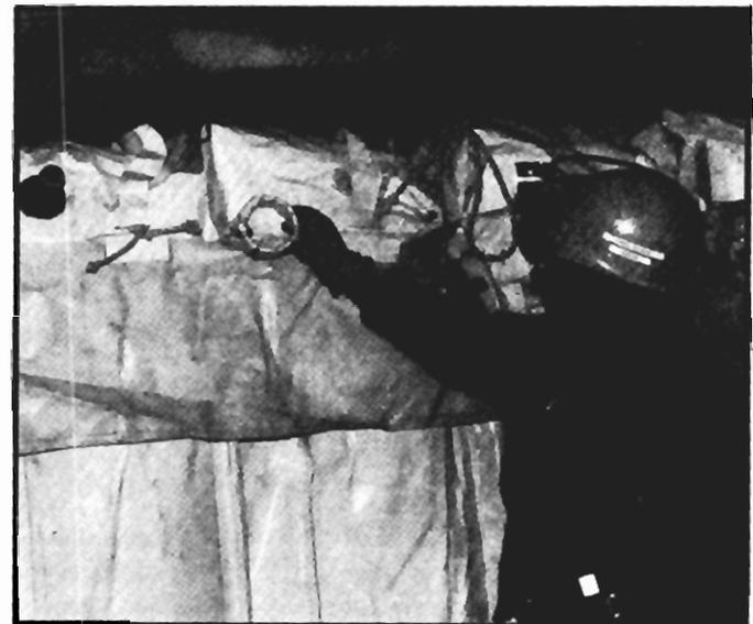
Figure 14.—Inflated vinyl bladder assembly showing the injection port for the piers.
