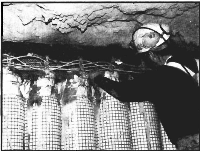
Figure 22.—Construction of seal in crosscut 4 showing details of the tops of the vinyl tubes and light meshing overlay.
