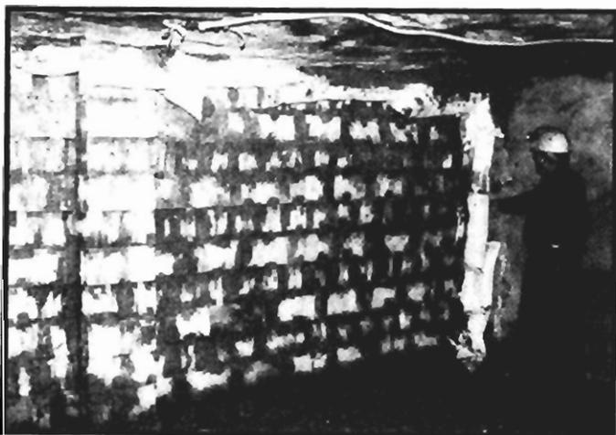
Figure 58.—Completed mortared seal with the Packsetter bags in crosscut 3.
