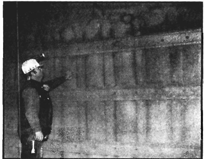
Figure 41.—Completed seal in the high roof section of crosscut 3.
