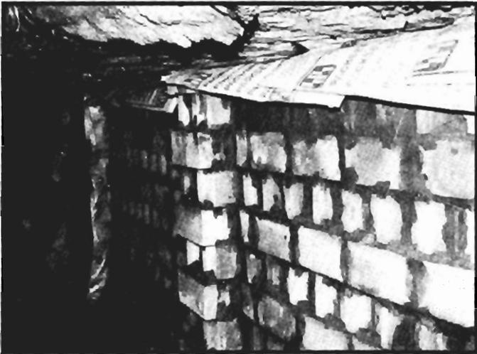
Figure 53.—Unfilled Packsetter bags at the seal interface with the mine roof and ribs.
