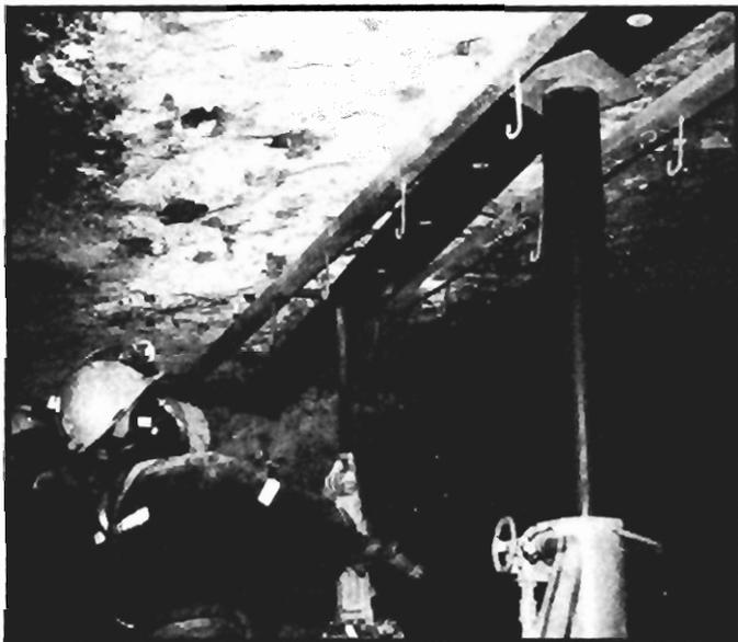
Figure 12.—Spreader bar anchored to the mine roof used to support the seal bladder system.
