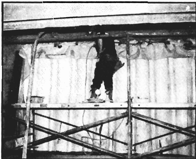
Figure 19.—Construction of seal in high roof section of crosscut 3, showing the grout injection hose attached to the bladder.
