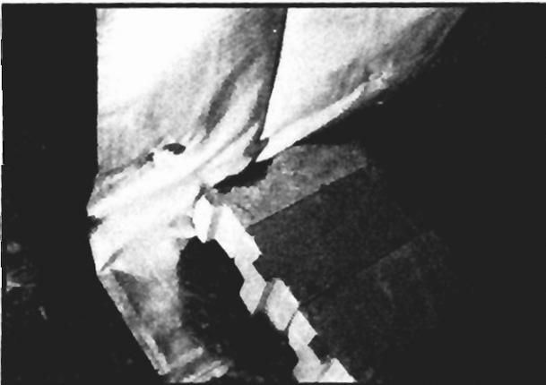
Figure 55.—Placement of the Packsetter bag at the mine rib and floor interface with the bottom course of the tongue-and-groove solid-concrete-block seal.
