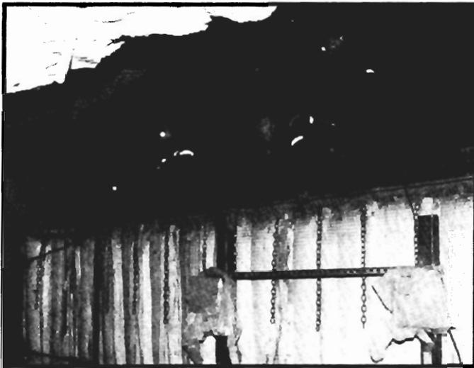
Figure 28.—Construction of overcast at the intersection of B-drift and crosscut 3: installation of skirt around edge of deck.
