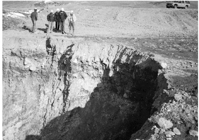
Figure 1.—Rock dump failure caused by water runoff.
