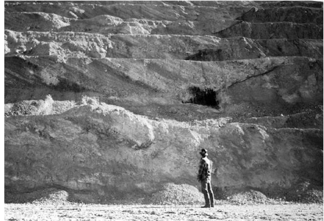
**Figure 2.—Rock dump with 15-m-high vertical benches.**
