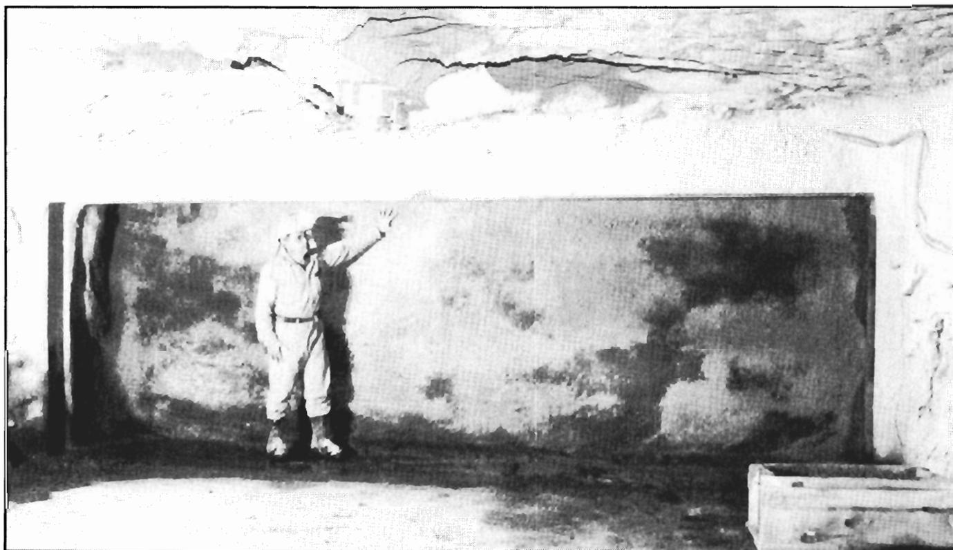
Figure 10.—Completed Meshblock seal in crosscut 2.
