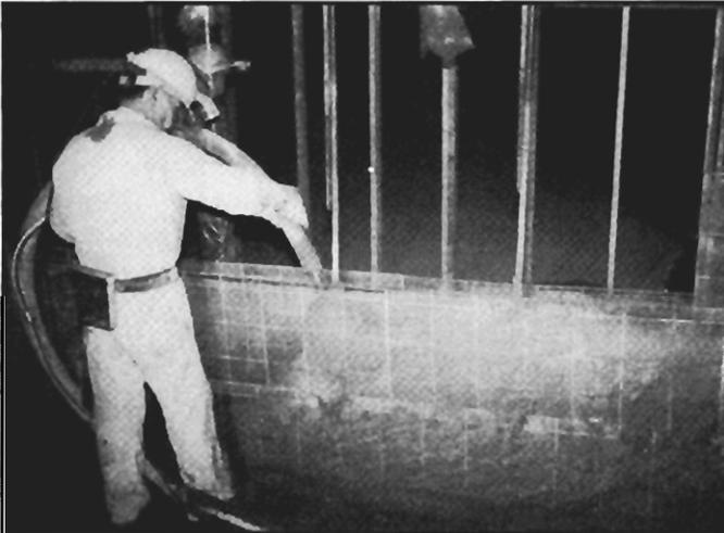
Figure 12.—Construction of Meshblock seal in crosscut 4.
