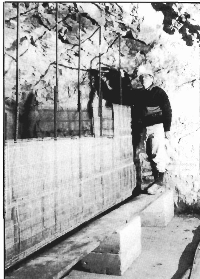
Figure 15.—Construction of Meshblock seal in crosscut 3, showing reinforcing bars anchoring it to the ribs and roof.
