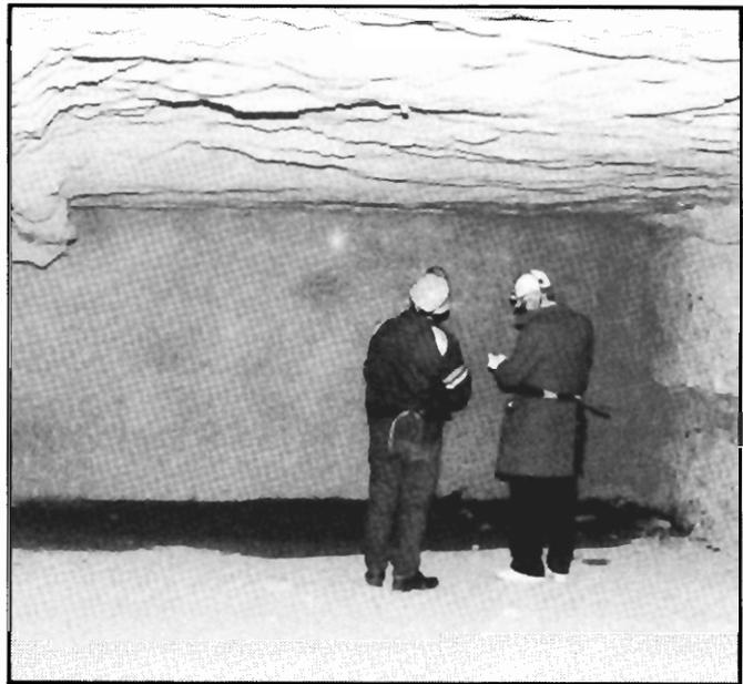
Figure 14.—Completed Meshblock seal in crosscut 4.
