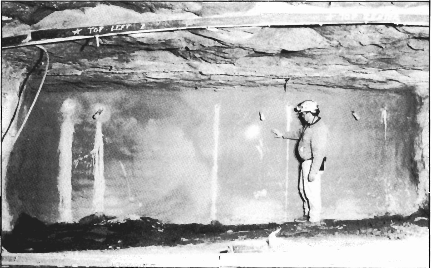
Figure 8.—Completed plug seal in crosscut 1.
