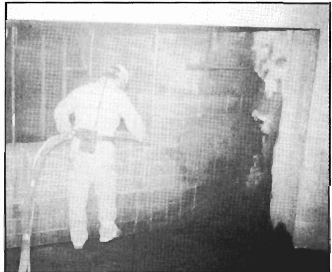
Figure 9.—Construction of Meshblock seal in crosscut 2.
