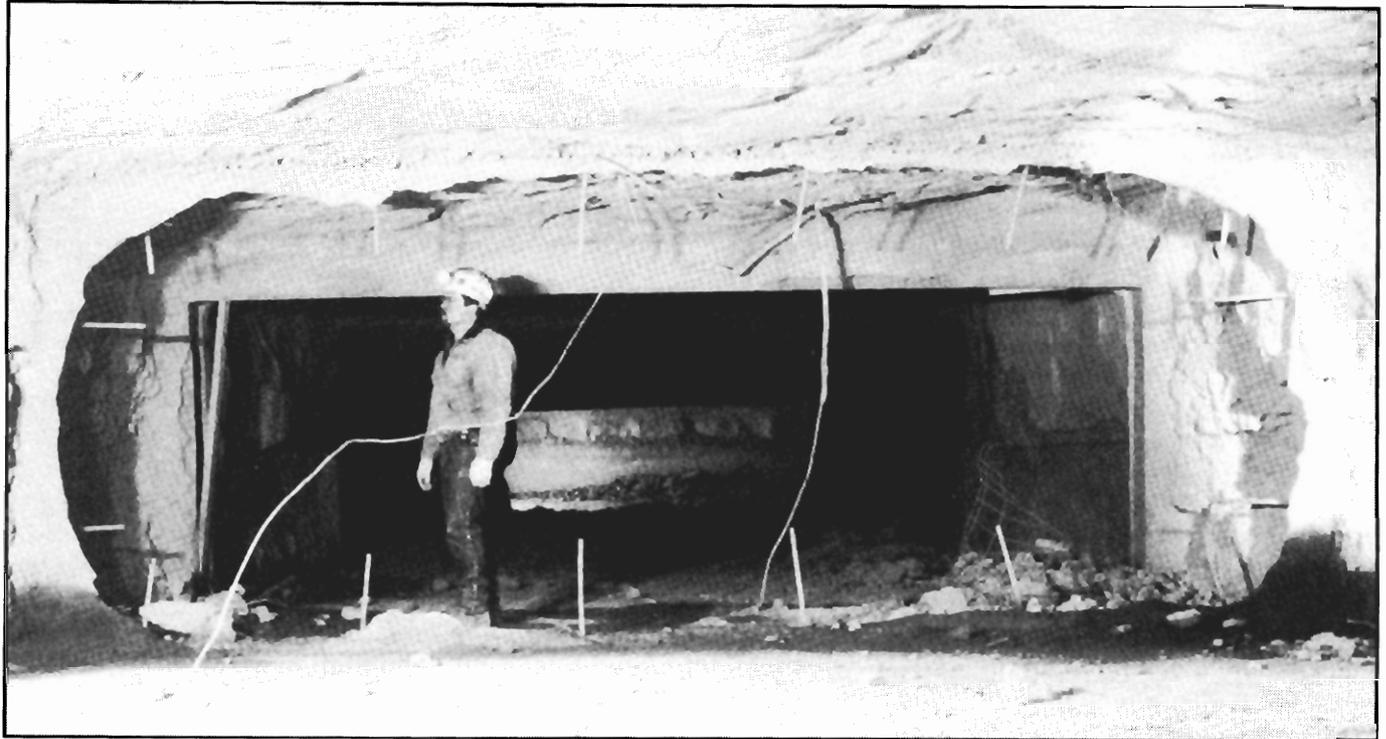
Figure 22.—Remains of stopping 5 after LLEM test 348.
