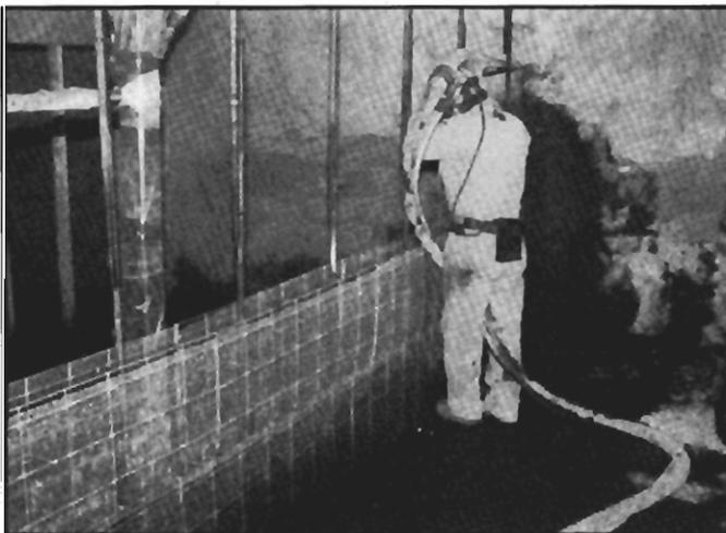
Figure 13.—Construction of Meshblock seal in crosscut 4.
