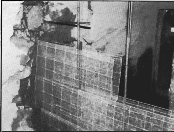
Figure 11.—Construction of Meshblock seal in crosscut 4, showing reinforcing bars anchoring it to the ribs and roof.
