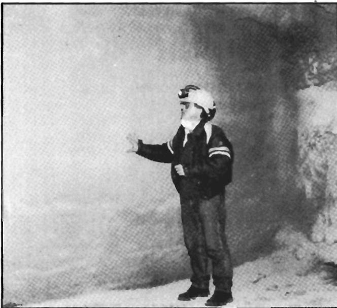
Figure 17.—Completed Meshblock seal in crosscut 3.
