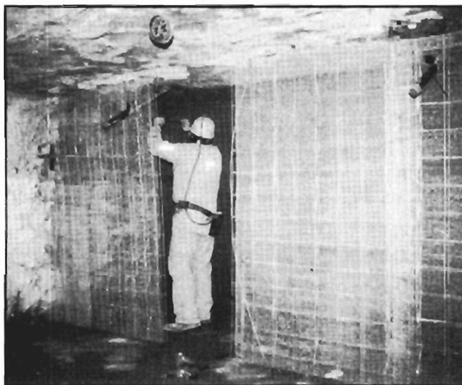
**Figure 7.—Construction of second wall of plug seal in crosscut 1.**
