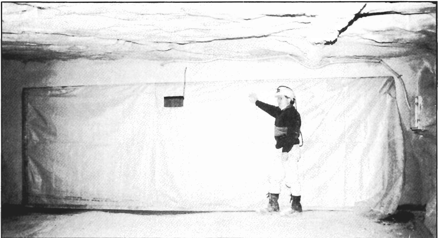
Figure 6.—Brattice in place for seal leakage test.
