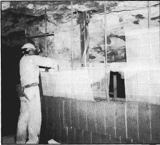
Figure 16.—Construction of Meshblock seal in crosscut 3.
