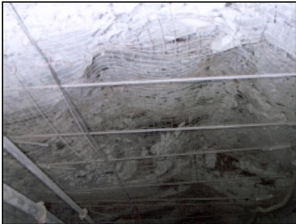
**Anomalous deformation of the roof might indicate an impending roof fall.**
