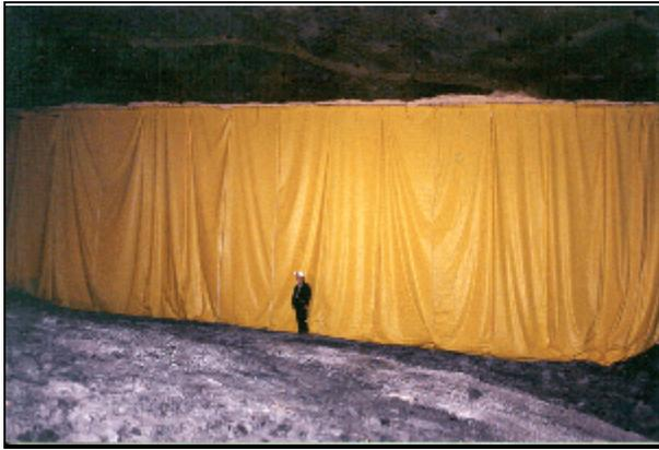
One of three brattice cloth ventilation stoppings installed in the Lake Lynn mine for this project.
