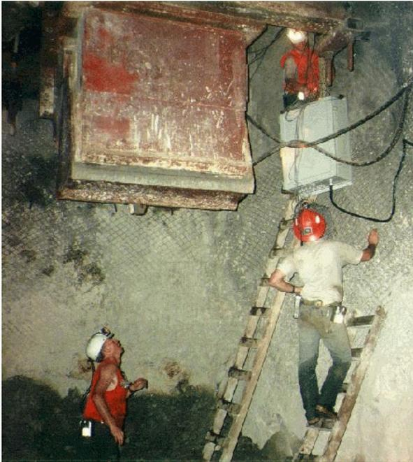
Loosening blockages in ore passes can be extremely hazardous.
