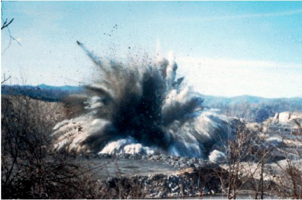
Flyrock being thrown by a surface blast.
