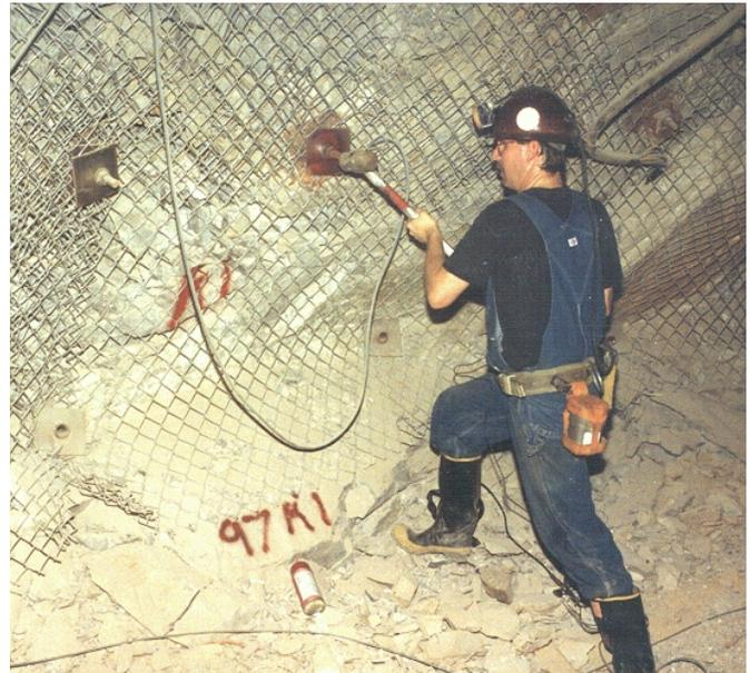
Figure 5.—Creating a source of seismic waves.
