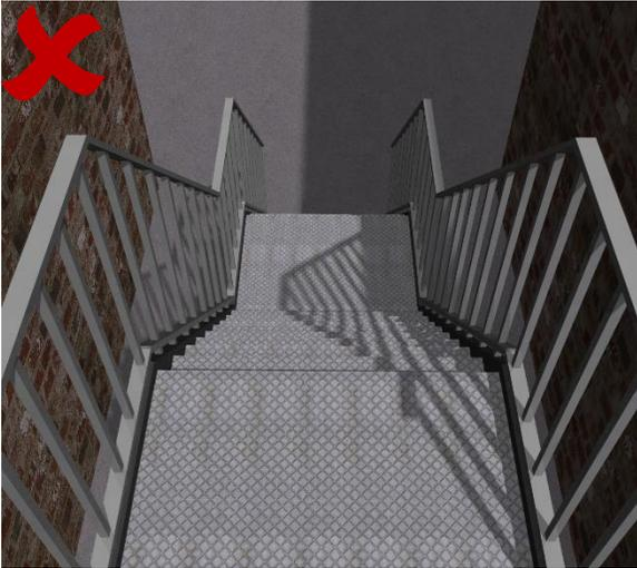
**Problem:** When the edge of the stairs (nosing) is not clearly visible, it can lead to trips, missteps, and falls.
