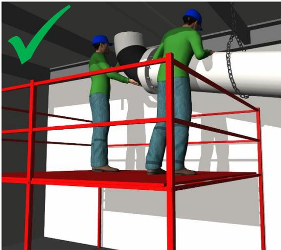
**Solution:** Supply scaffolding when multiple people are working on elevated objects. Care must be taken to ensure that workers are not situated above the highest level of the scaffold and that the platform is guarded on all sides. If scaffolding is designed and used appropriately, it can also eliminate the need to use personal fall protection.
