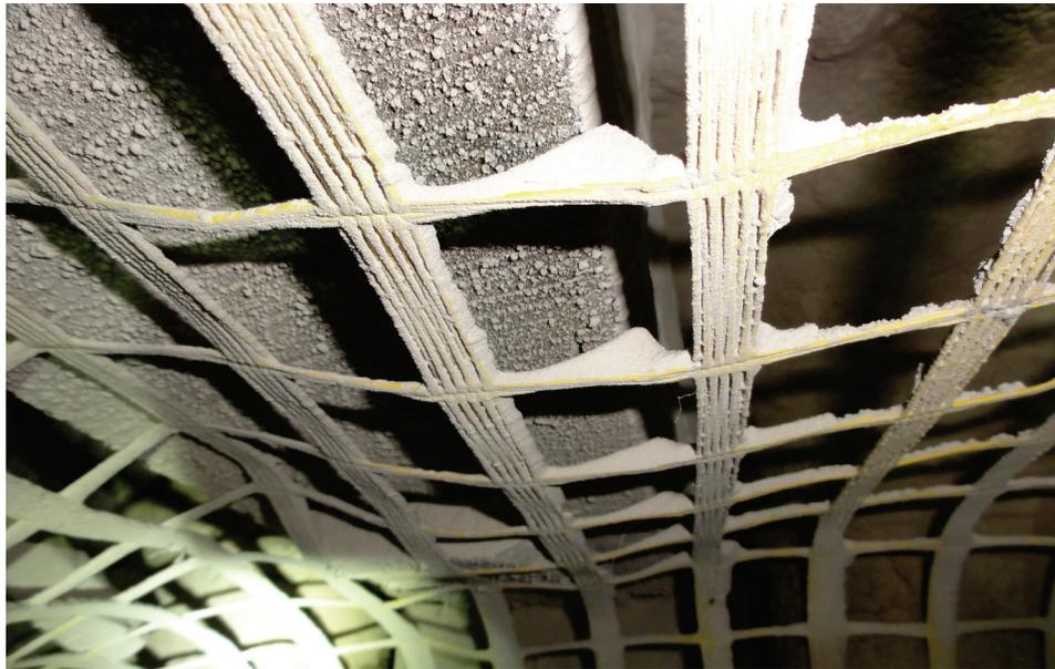
**Figure 10. Indirectly applied rock dust is visible on the elevated surface of the mesh.**
