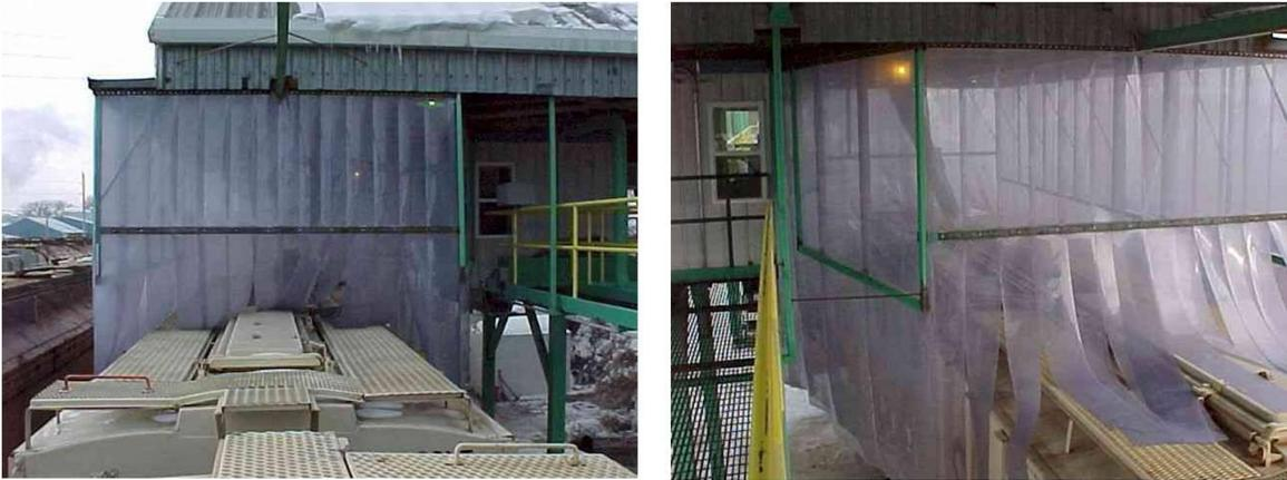
**Figure 7.7. Rail car loadout area enclosed with plastic strips to contain dust.**
