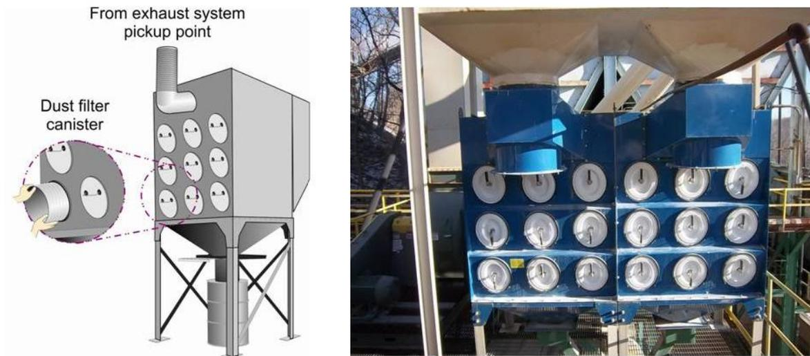
**Figure 1.20. Cartridge collector with dust filter canisters.**
