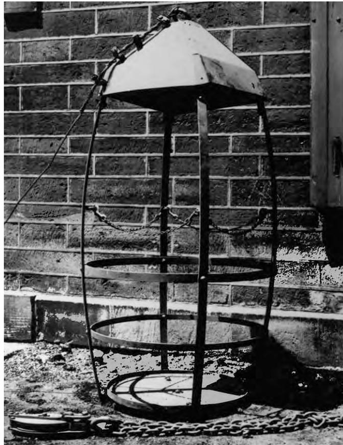
**Figure 19.** Collapsible cage used for mine rescue.
